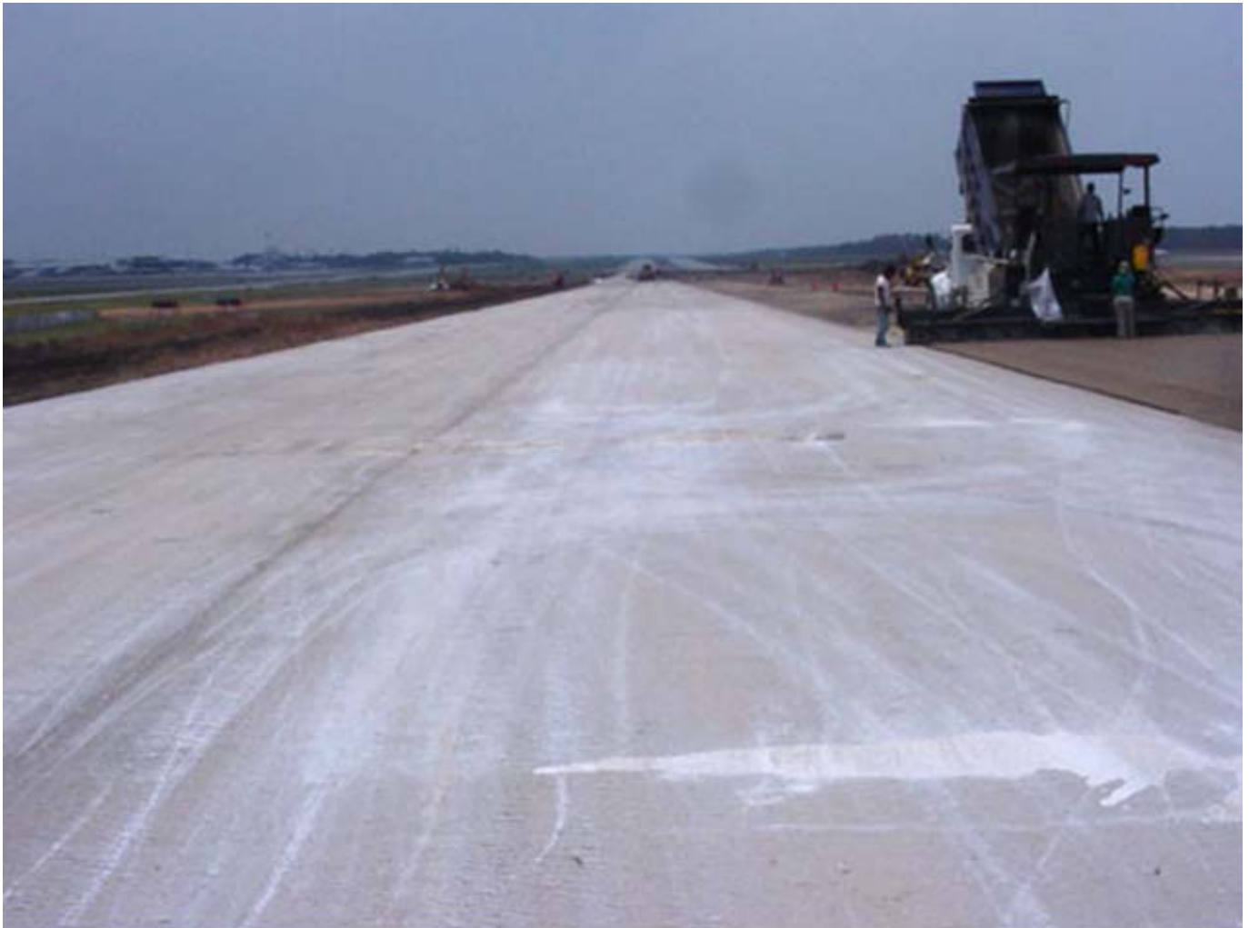
Photograph of Cement Stabilized Roadbed
